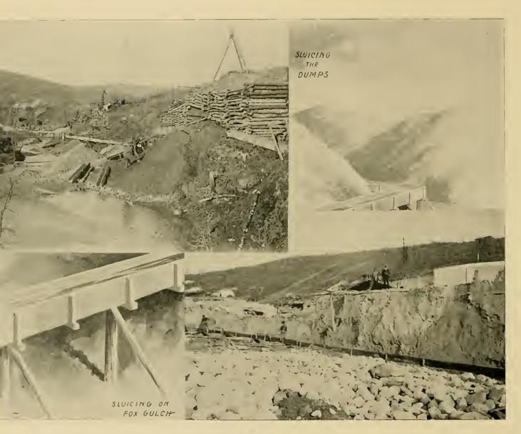
ALL PLACER GOLD IS RECOVERED FROM THE GRAVEL BY SLUICING
