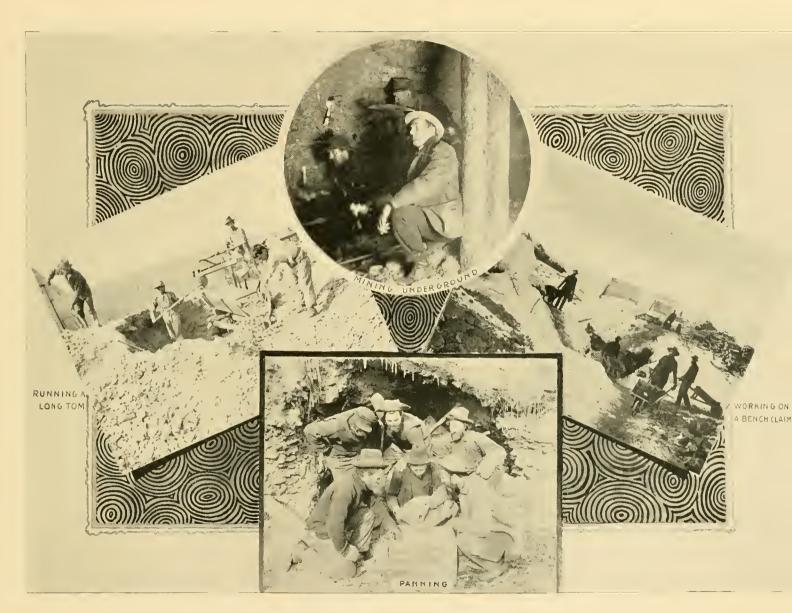
THE GOLD PAN IS SYMBOLICAL WITH PLACER MINING AND IS INDISPENSABLE IN TESTING THE VALUE OF GRAVEL
