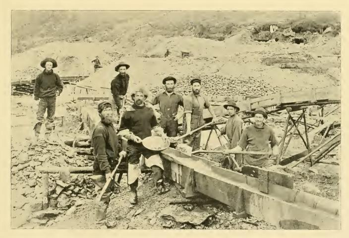
IN KLONDIKE, PREPARATORY TO SLUICING, THE GRAVEL IS MINED FROM THE CREEK BOTTOMS AND HIGH BENCHES-THE YEAR AROUND THE GROUND IS FROZEN AND MUST BE THAWED
